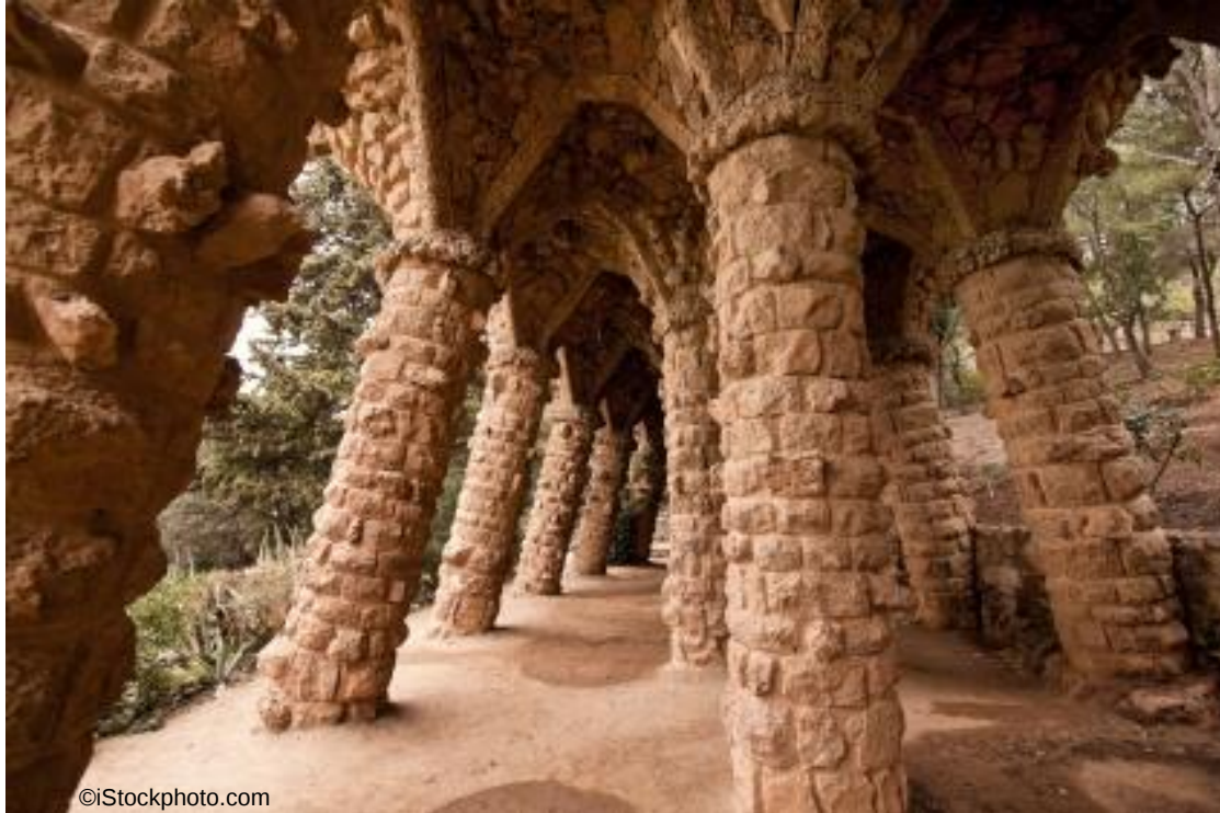
Park Güell – Barcelona, Spain Architect: Antonio Gaudí
