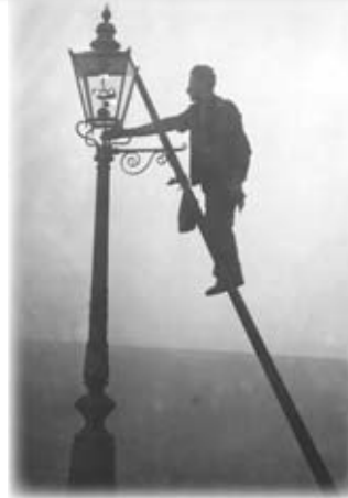
Gaslights were dangerous.
