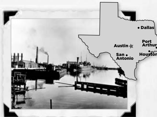
Port Arthur was known for its huge oil refining plants.
